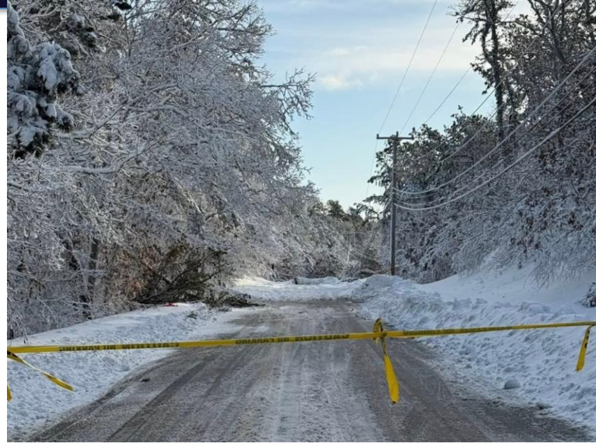
Damaged power lines in Brewster, MA from February 24, 2026 (masslive.com)
